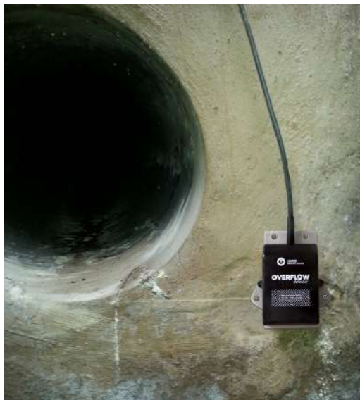
Installation in storm drain
