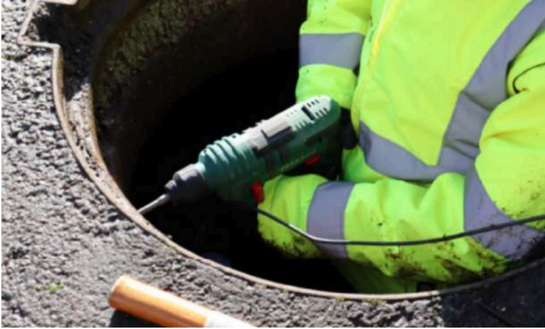
Drilling into the manhole
