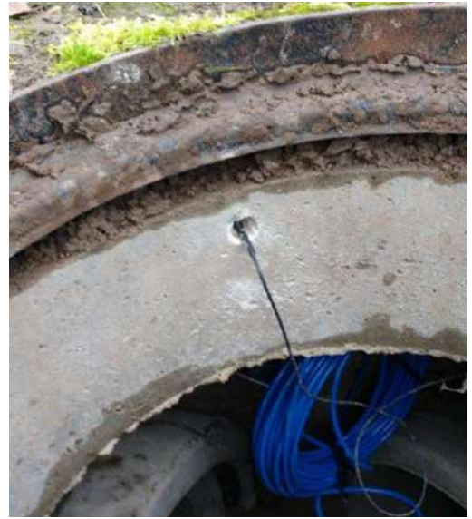
Inserting antenna under the base
