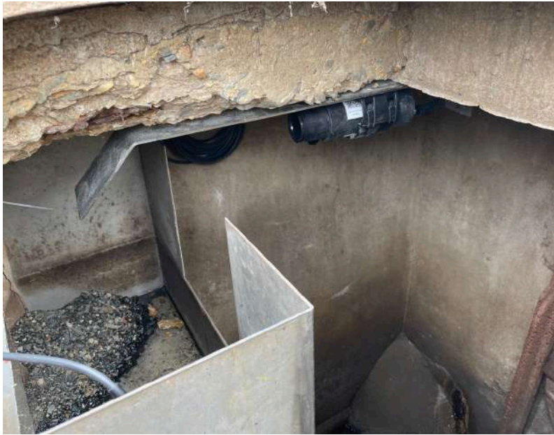
Installation with angle rebate mounting kit
