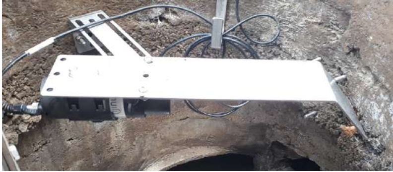
Installation with angle rebate mounting kit
