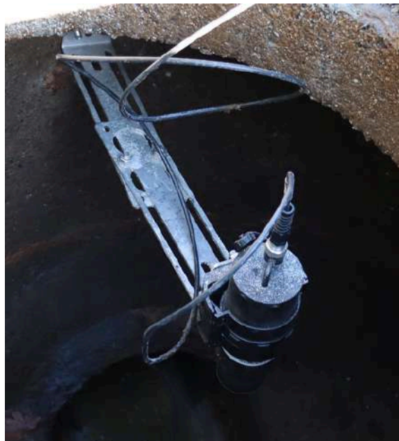
Example of installation with two mounting plates
