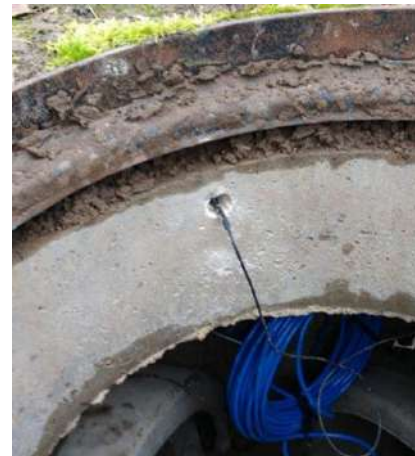
Inserting the antenna under the sole
