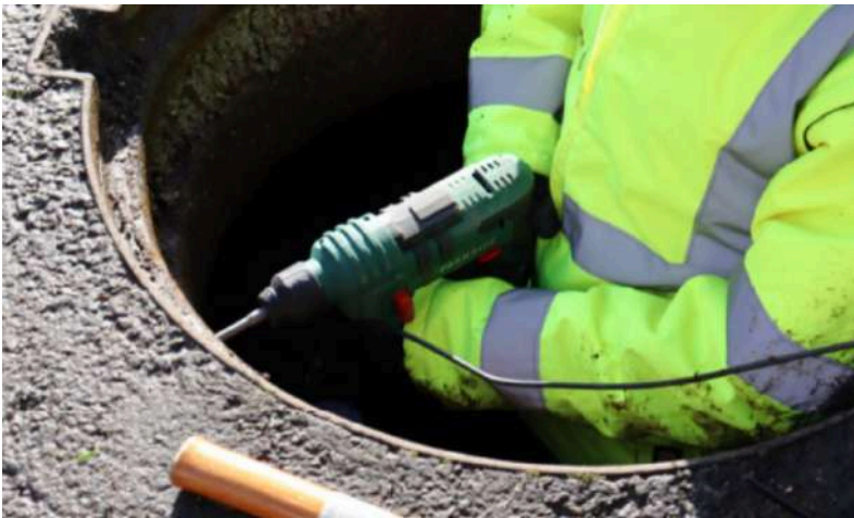
Drilling into the manhole
