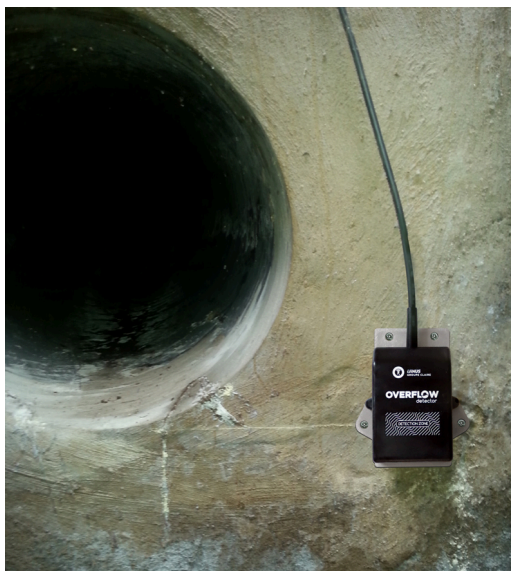
Installation in storm drain
