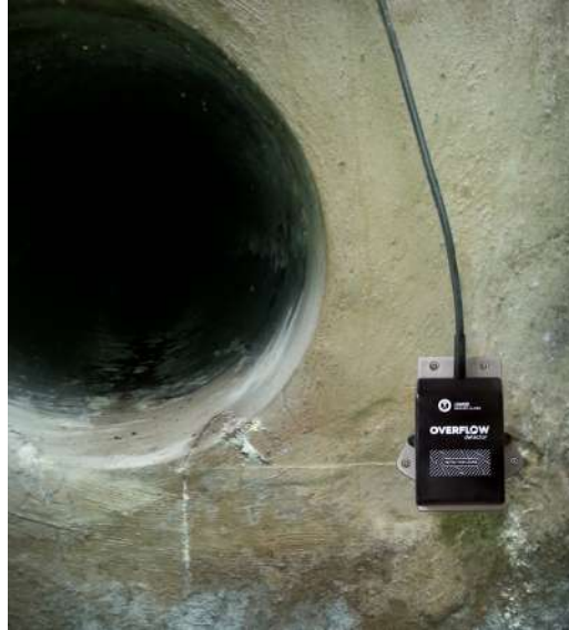
Installation in storm drain
