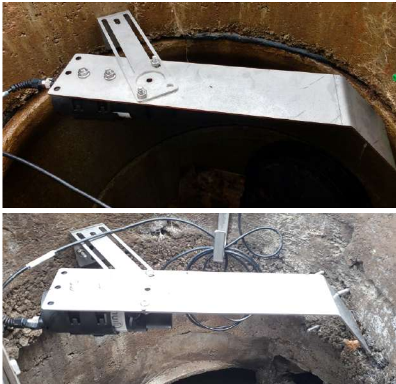
Installation with angle rebate mounting kit
