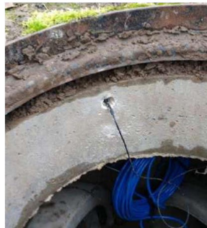
Inserting the antenna under the sole
