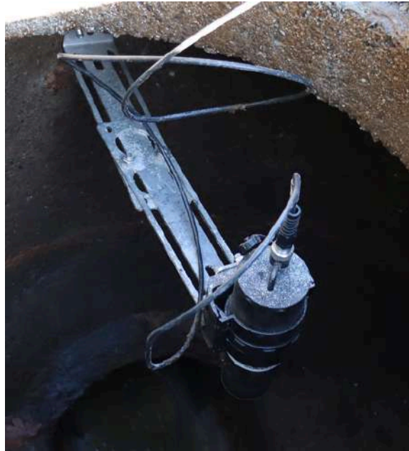
Example of installation with two mounting plates
