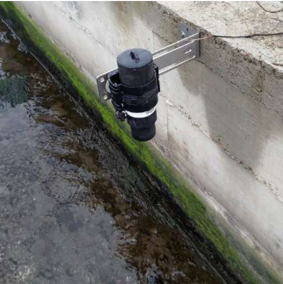
Example of installation with a mounting plate
