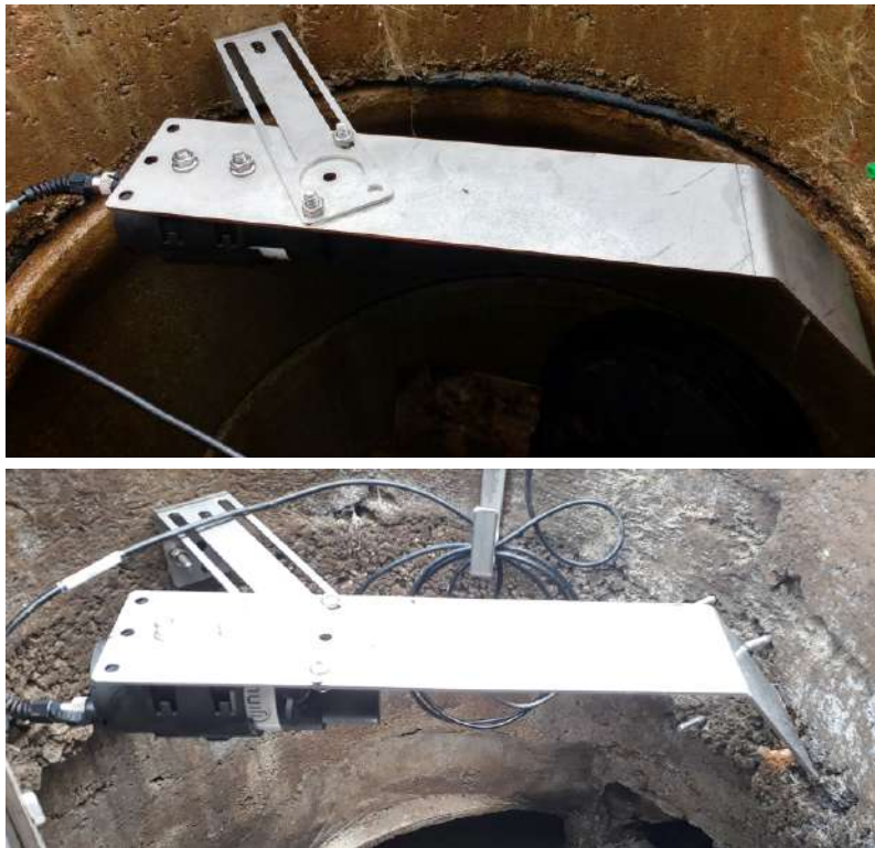
Installation with angle rebate mounting kit
