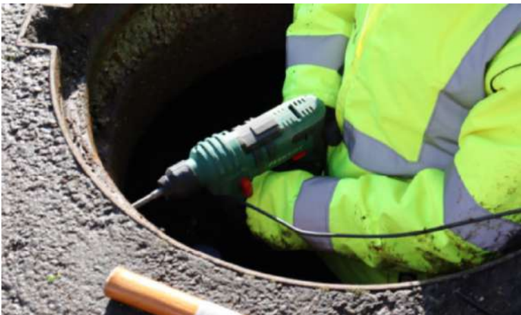
Drill hole in manhole
