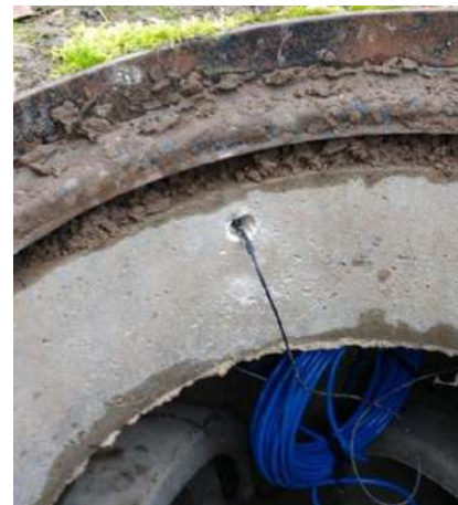
Inserting the antenna under the sole
