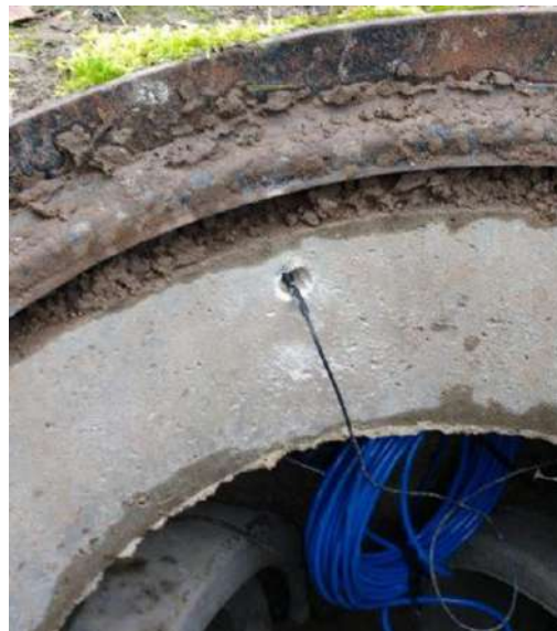
Inserting antenna under the base
