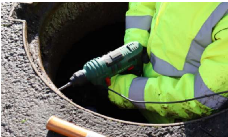
Drilling into the manhole
