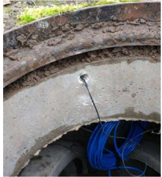
Inserting antenna under the base
