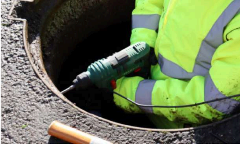
Drilling into the manhole
