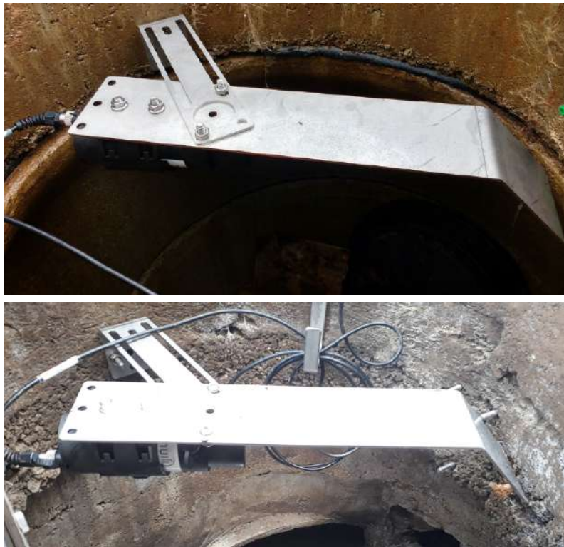
Installation with angle rebate mounting kit
