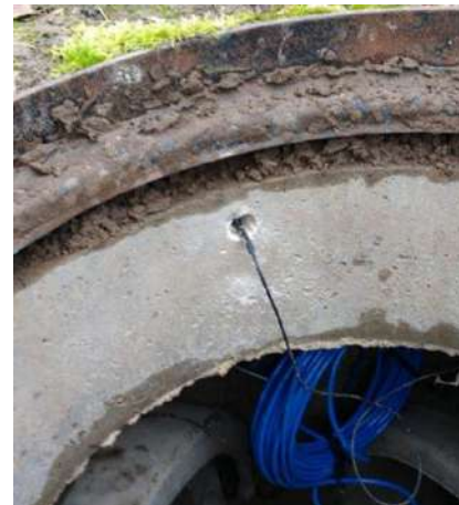
Inserting the antenna under the sole
