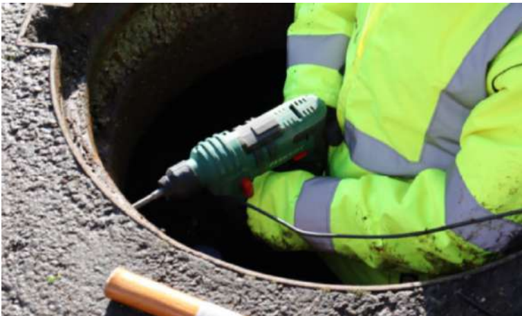
Drill hole in manhole
