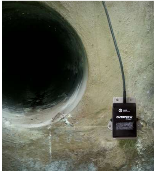
Installation in storm drain
