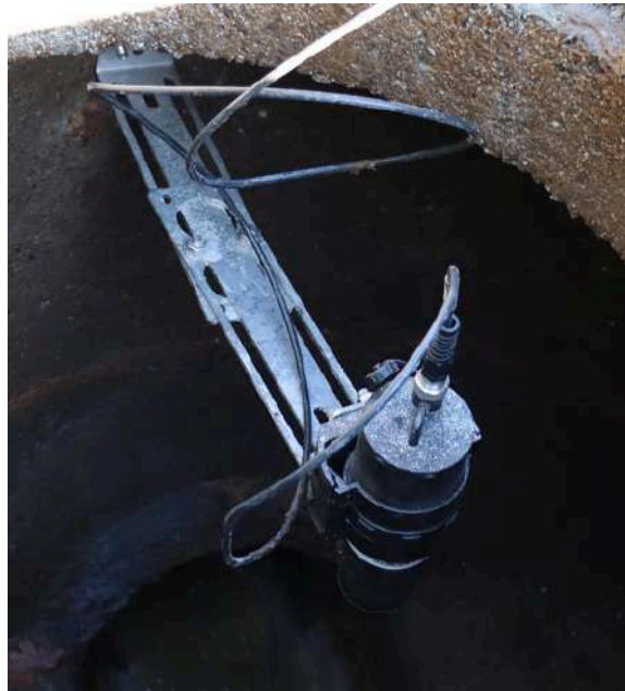
Example of installation with two mounting plates
