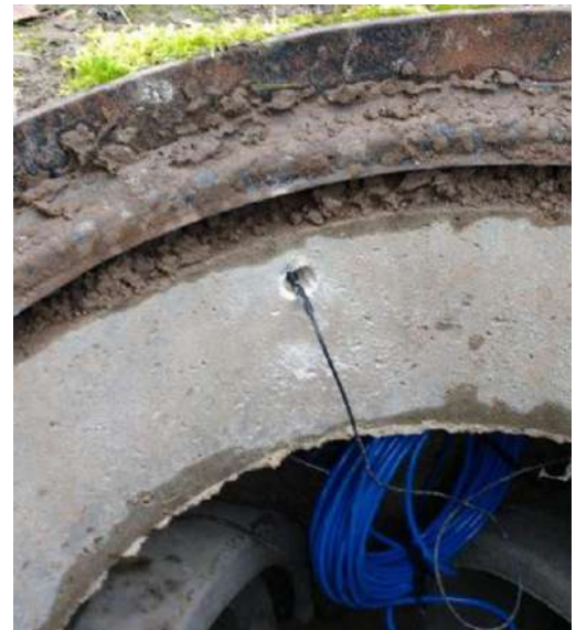
Inserting antenna under the base
