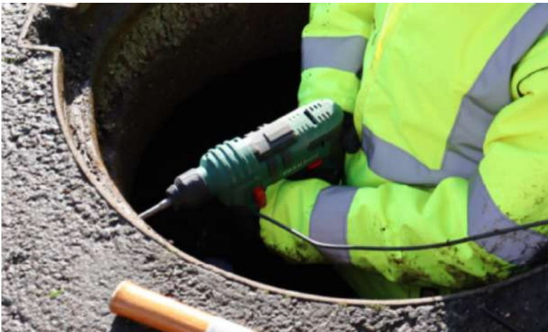
Drilling into the manhole
