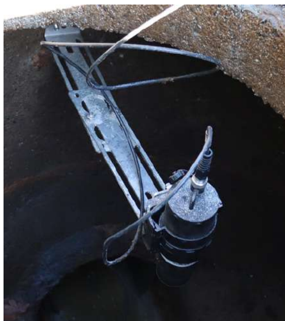
Example of installation with two mounting plates
