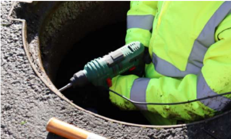
Drilling into the manhole
